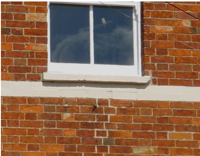
Rear garden of Wymering House. Asterisk shows the point of entry of the bomb. The damage to the sill and the area of repointed brick-work are still just visible in the close-up below.
