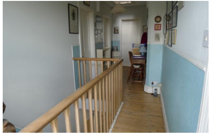
The top landing via which the bomb travelled on its way to the door of the storage room at the end. The bannisters are modern replacements.
